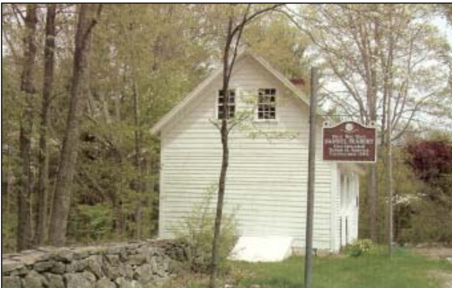
Gurdon Bill's Station, Ledyard, CT. This Country Store and Stagecoach Way Station dates from 1816
